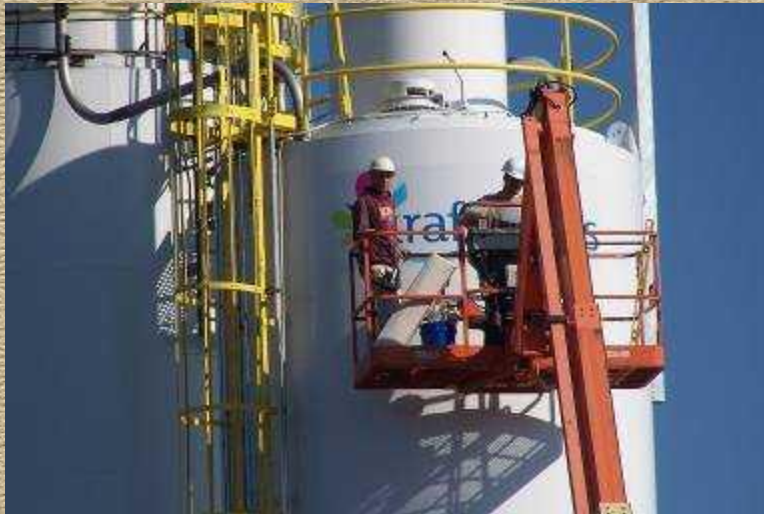
Sign installation in progress
