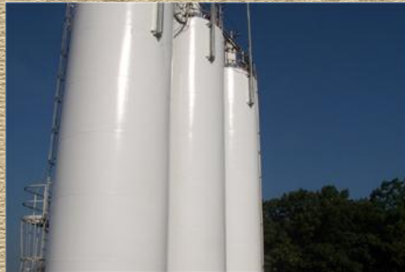
Image of silos with fluorourethane finished coating installed
