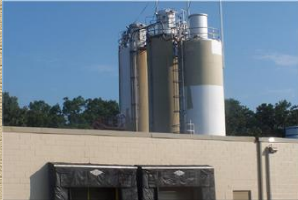
Progression image of silos being coated with polyamide epoxy base coat
