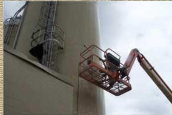
Additional image of water blasting prior to coating install
