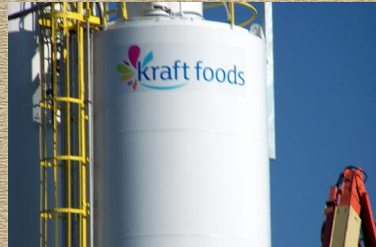
Completed sign installation on silo one
