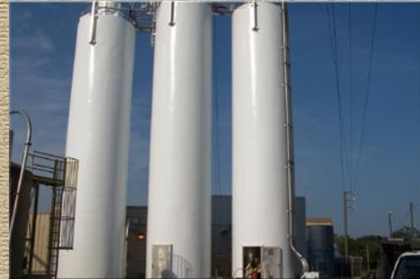
Image of silos completed with polyamide epoxy base coat
